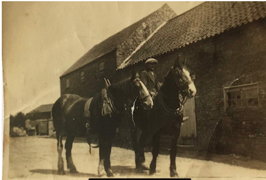
The barn between 1930 and just after WW2 before it's restoration (as shown in the photo above).
